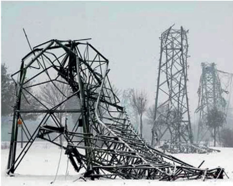
Figure 6: Extreme ice and snow loads on pylons near Münster, Germany in autumn 2005
